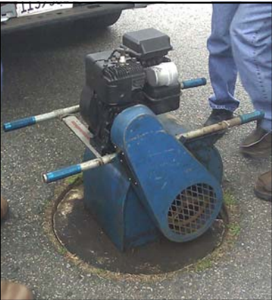
Gas-powered blower positioned over manhole access to sewer line.
